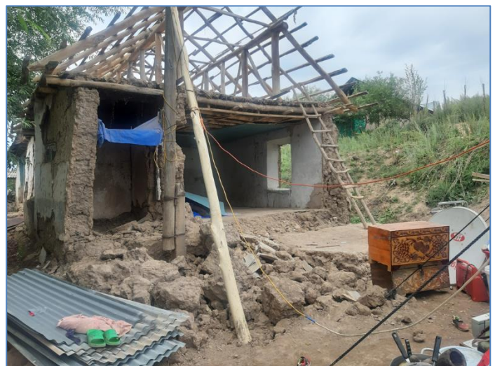
Destroyed house in Buston, Tajikabad district Photo credit: OCHA
