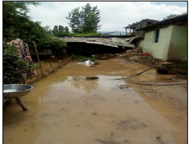
Damaged house in Rudaki District. 1 June 2019. Photo credit: RCST
