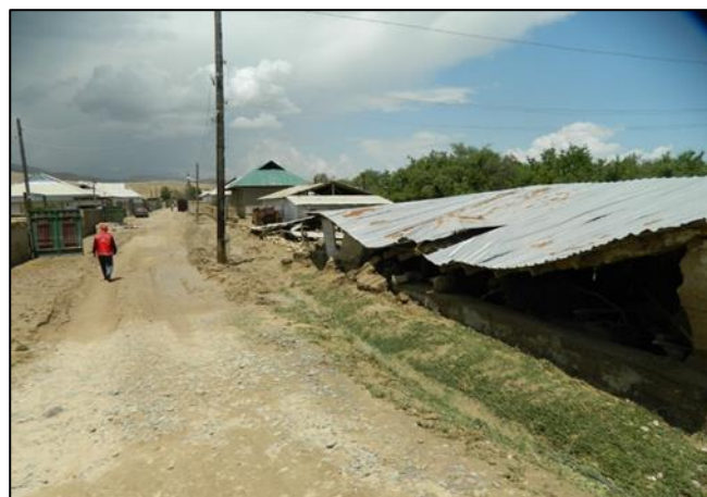
Damaged house in Khuroson District. 2 June 2019. Photo credit: RCST
