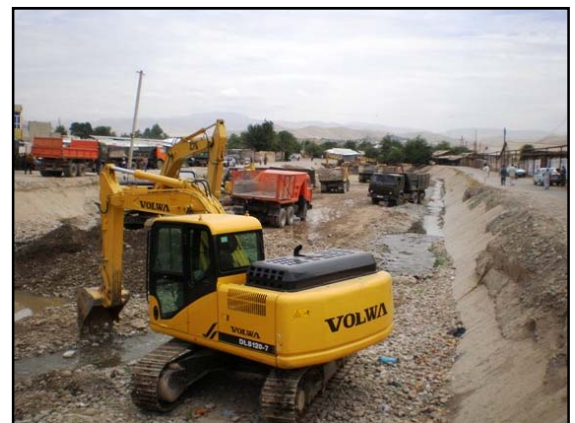
Photo 1: Cleaning of the Tebolay Channel
