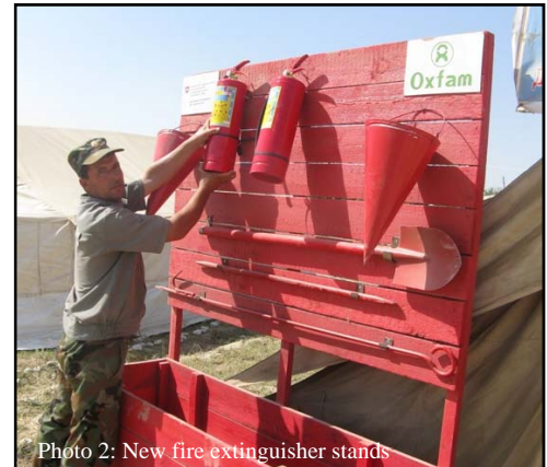
Photo 2: New fire extinguisher stands
