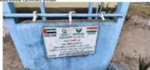
Water Tap at the Medical Centre Compound
