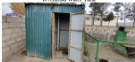
Existing Toilet Facilities
