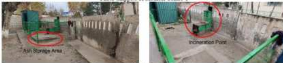
Waste storage and incineration (Local) point
