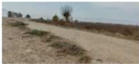
No shoulder/footpath on the road
