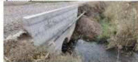
Canal passes through the Bridge-1
