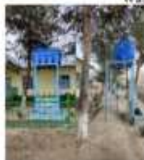
Overhead Water Tank
